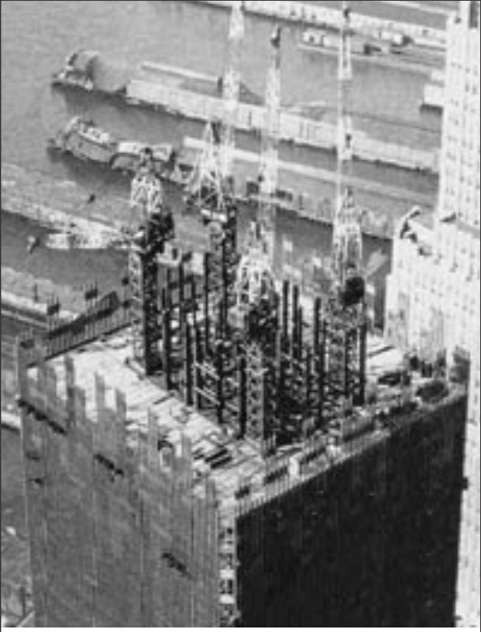
This photograph of World Trade Center construction reveals the massive central core of the building.
