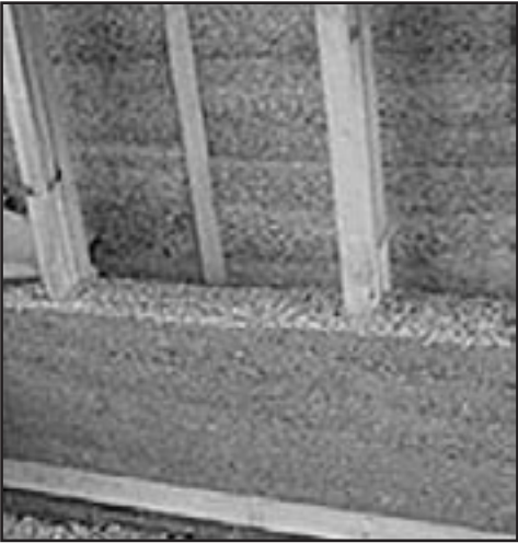
Close-up of hemp wall construction.
