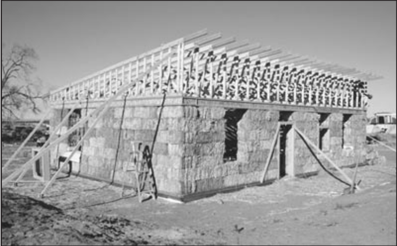
Construction of a straw bale home in Hotevilla, Arizona.
