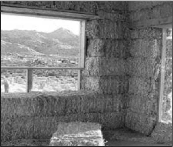
Unfinished interior wall of straw bale B&B in southeastern California.
